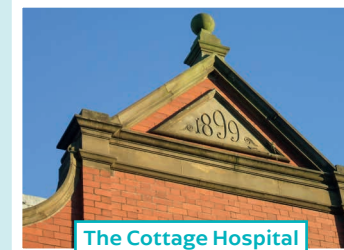
The Cottage Hospital extension
